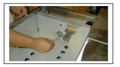
2-6) Remove the LP Hose and Regulator Assembly from the coupling, and remove the 3/8 Flare x 1/2" FIP coupling by turning the coupling counter-clockwise with an adjustable wrench.
