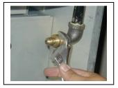
2-7) Install the factory supplied Natural Gas regulator directly to the manifold and use pipe sealant approved for natural gas connection. Use a 12" Adjustable Wrench to turn the regulator and a Pipe Wrench to hold the manifold in place. Warning: The Natural Gas Regulator is set at 4" of Water Column.
